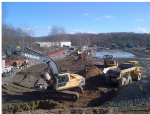
The Mark I Fairfield County will feature 228 units when completed next year.
